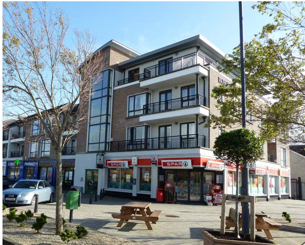
Modern shop front with corporate signage
