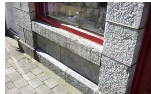
Stone stall riser to premises along High Street
