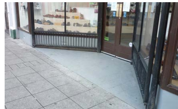
Views of thresholds & lobby set backs. In some cases with historic structures level entrances are not practicable.
