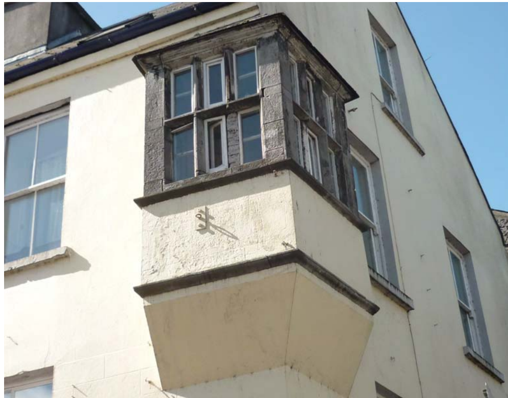
17th C. projecting window to corner of Cross Street & Quay Street
