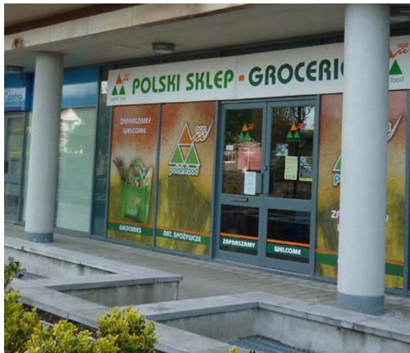
Shop front to modern development with excessive signage
