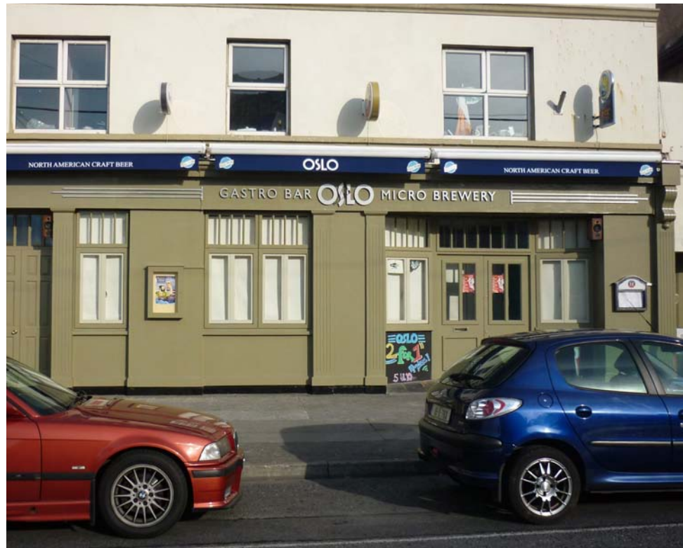
Good quality contemporary shop front using traditional details
