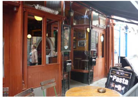
Rare example of historic timber shop front
